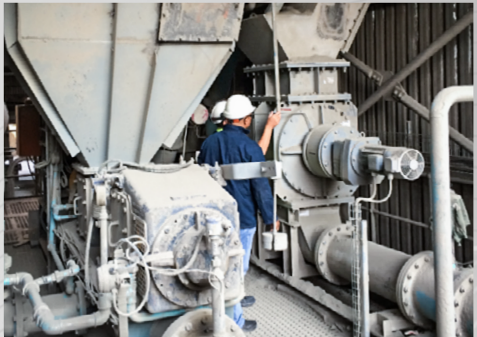
Exchange of Screw pump against KREISEL ceramic rotary feeder
